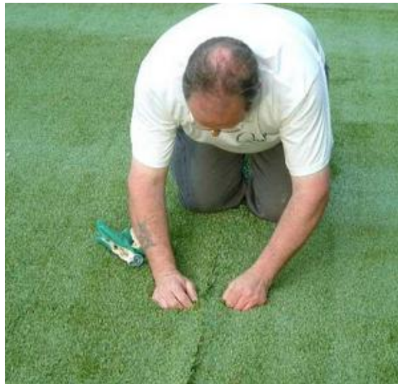
Laying Artificial Lawn Turf - Step 7 Dressing the grass
