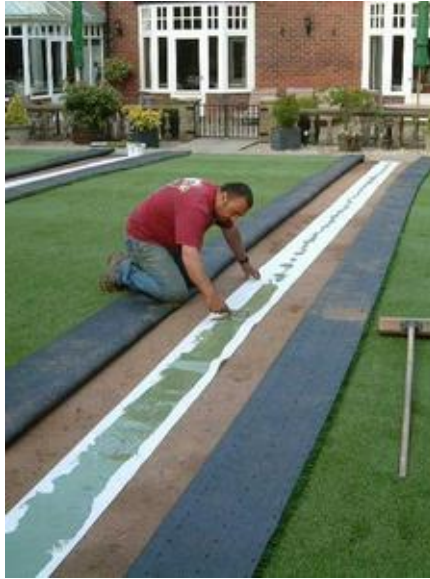
Laying Artificial Grass Guide - Step 6 continued
